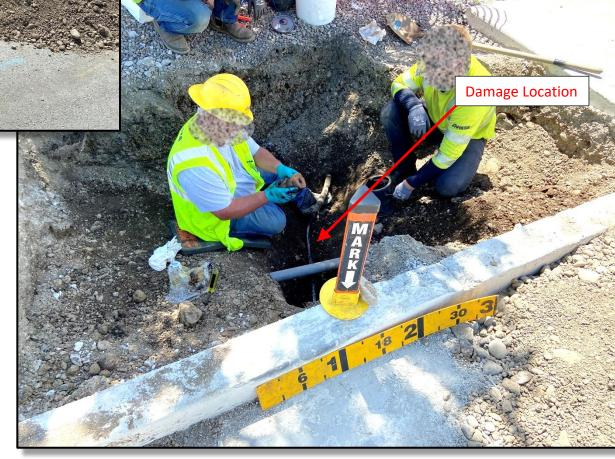
**8. Depth of Utility** – Shows there was roughly 20 inches of dirt cover for the gas line below the bottom of the sidewalk panel.
