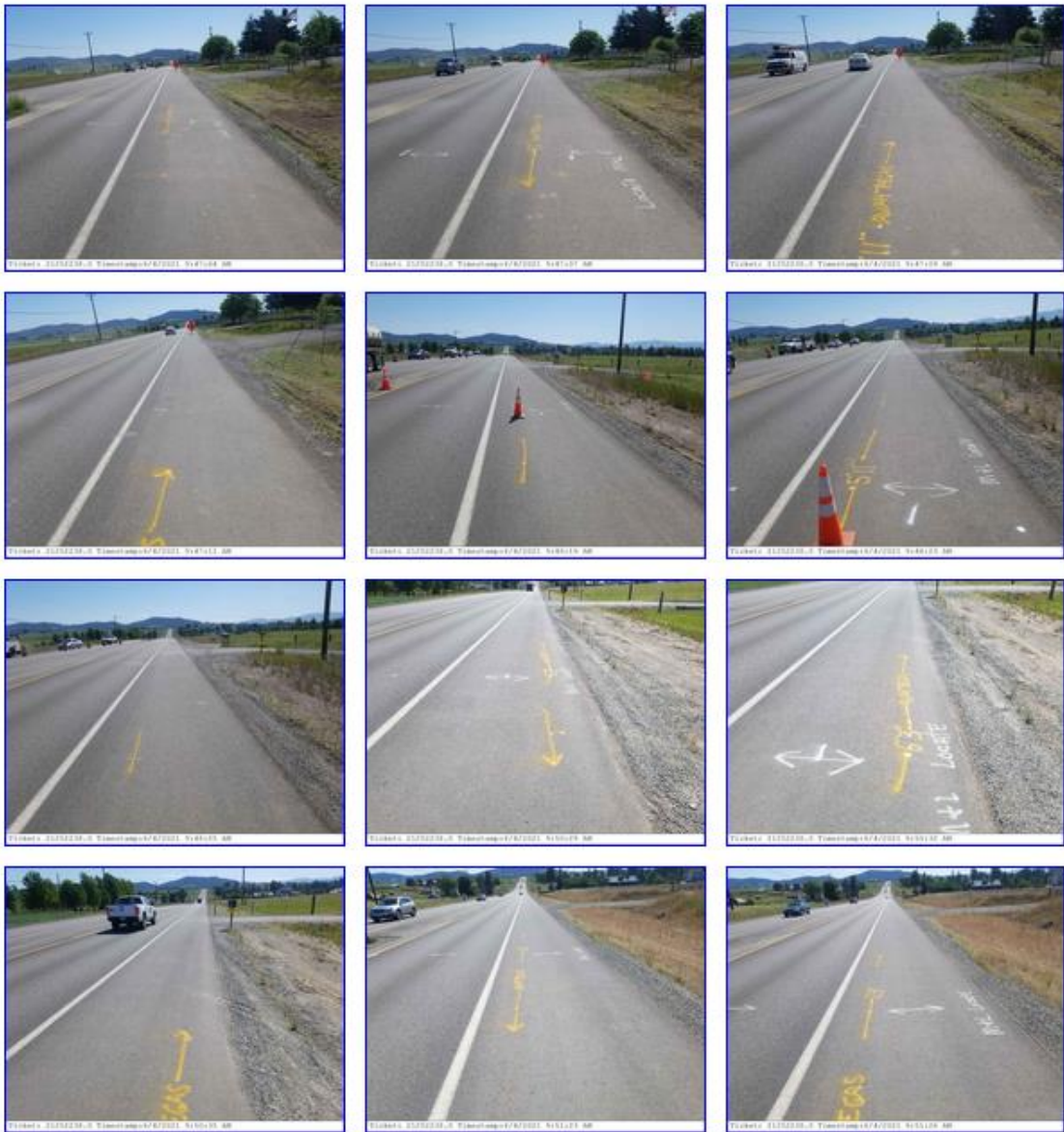
Exhibit D – Photos of locates performed on 6/4/21 indicating the 4" pipeline in the south shoulder of the road.
