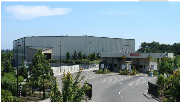
Airport Road Recycling and Transfer Station
