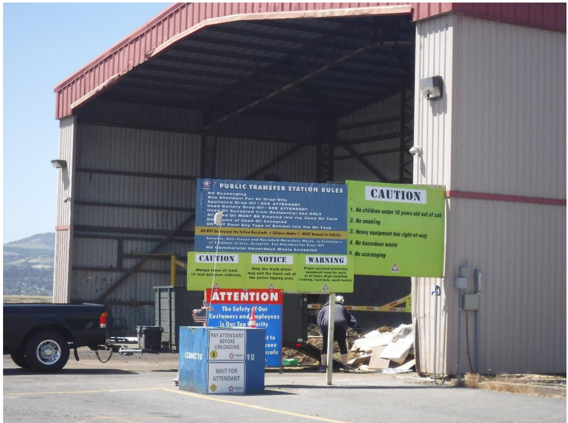
Figure 6-2. Dallesport Transfer Station
