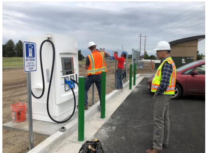
DCFC site construction at the West Plains Transit Center and Park & Ride—in partnership with Spokane Transit Authority (2018)
