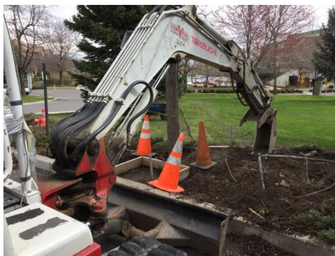
AC level 2 EVSE site construction in partnership with WSU (Riverpoint Campus, 2017)
