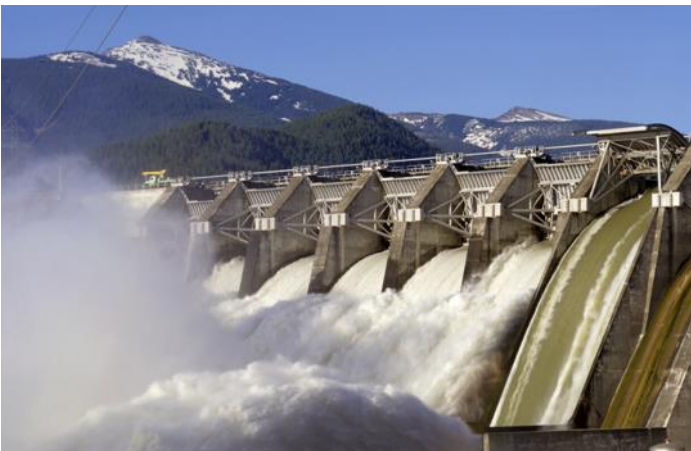
Avista's Noxon Rapids Hydroelectric Generation Plant – 562 MW of Clean Hydropower –
