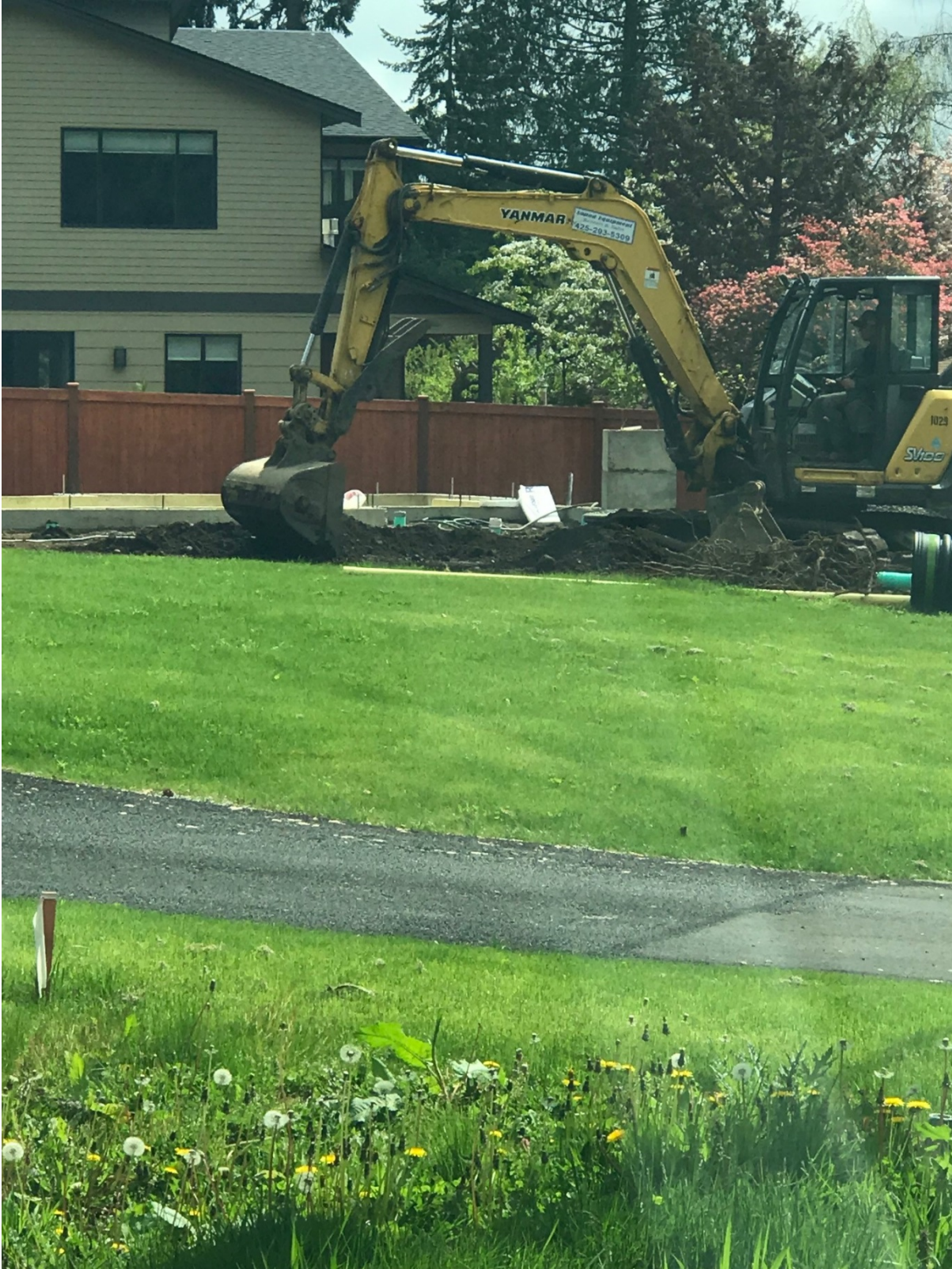
Excavation on site
