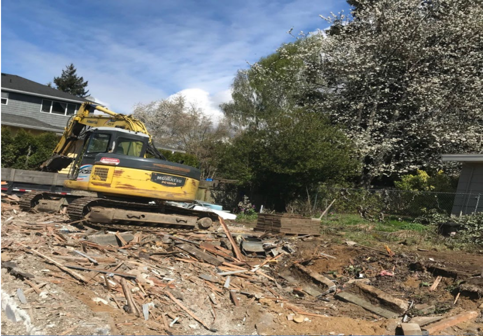
Two pictures of machinery onsite in the demo area:
