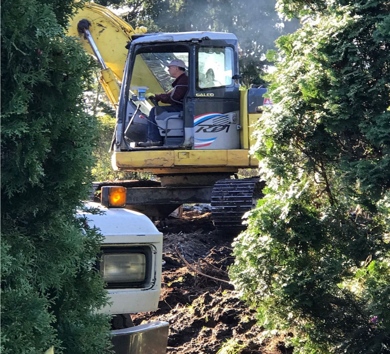
Pictures of active excavation:
