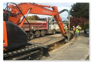
in established municipal areas neighborhoods with existing paved roadways, sidewalks, landscaping, and underground other facilities. The illustration at left shows the pavement cut required for open trench installation of new main pipe.
