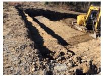
• In this series of three pictures Wallin Excavating has established the rough elevations of the foundation. The center picture shows one of Wallin Excavating's employees with a measuring rod.
