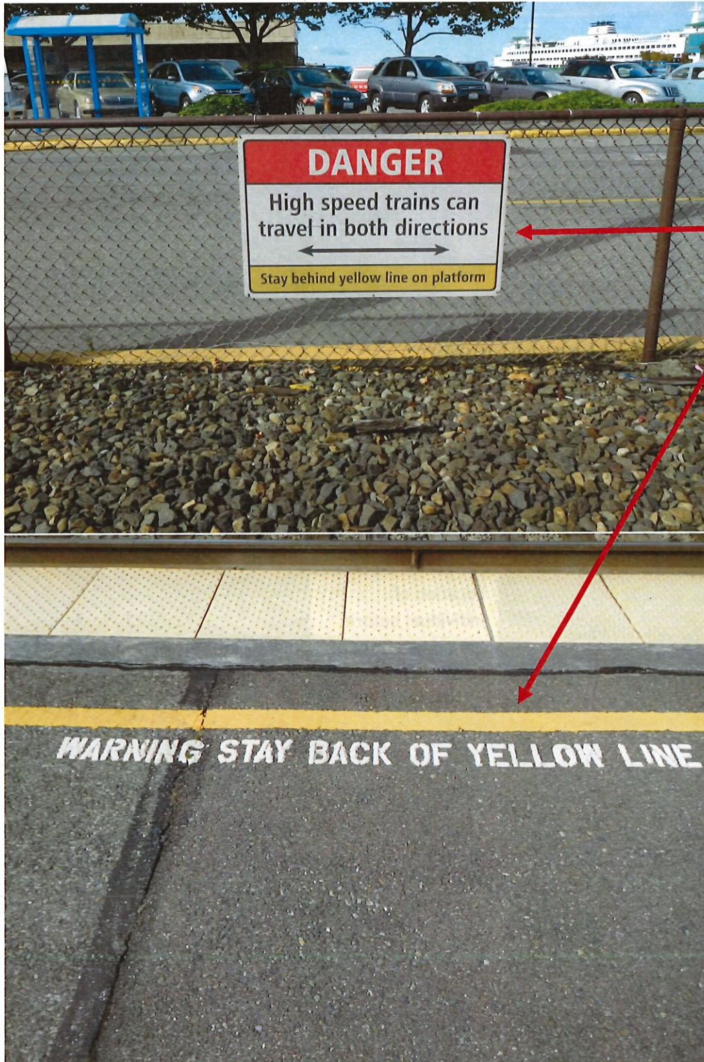
Signs warning of high speed trains and yellow line painted on passenger walk path
