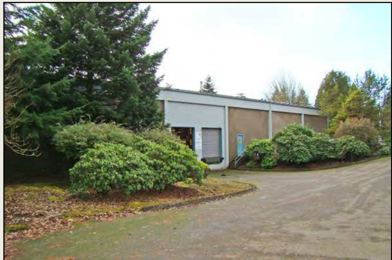
Photo 5: Facing west toward the Building B loading docks from McEwan Road
