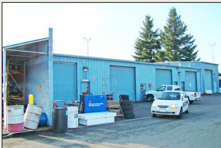
Photo 13: Facing west toward Building C
