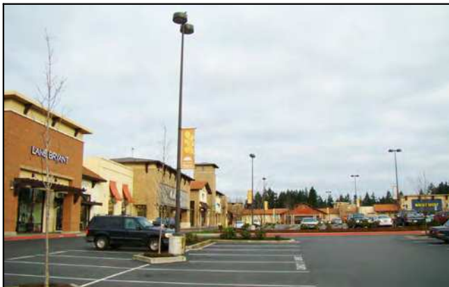
Nyberg Woods, located at the northeast corner of the intersection of I-5 and Nyberg Road
