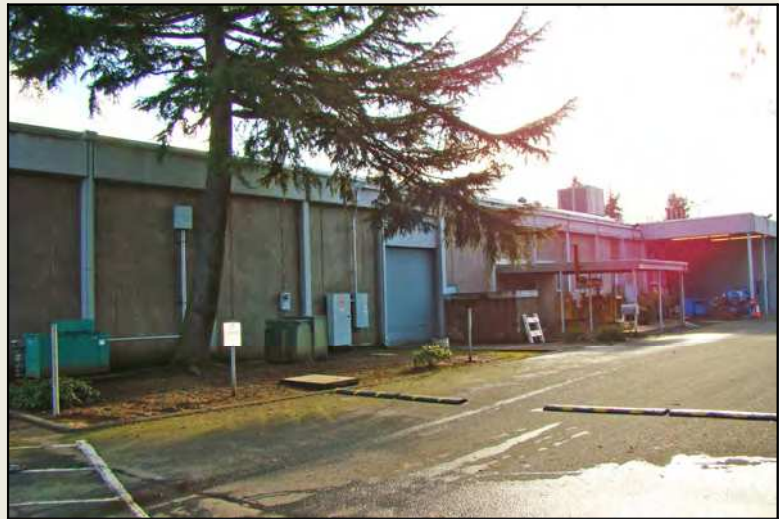
Photo 7: Facing south toward Building A
