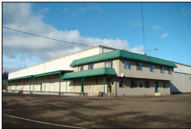
10655 SW Greenburg Road, back building
