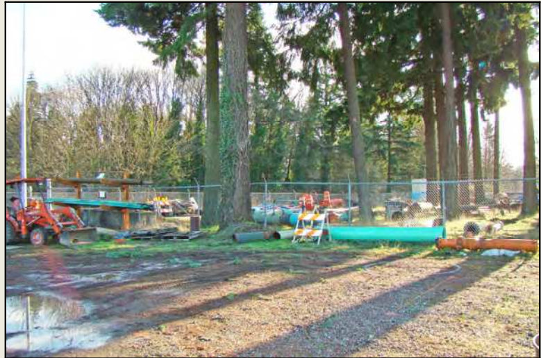
Photo 17: Facing south toward the bio swale area
