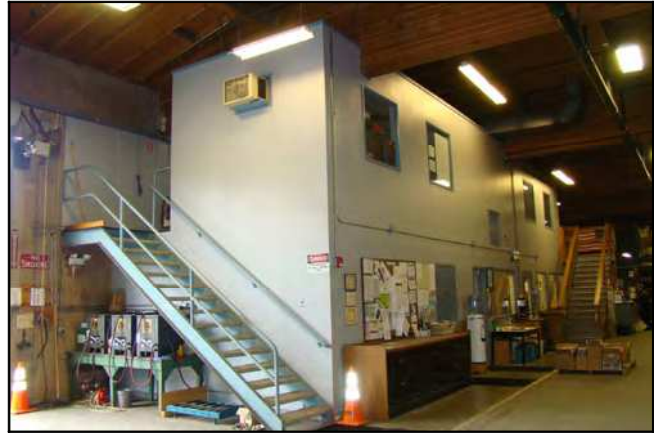
View of the Building B office space from within the warehouse
