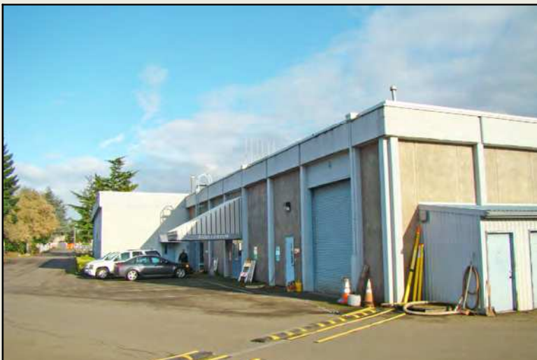
Photo 12: Facing east along the front of Building A
