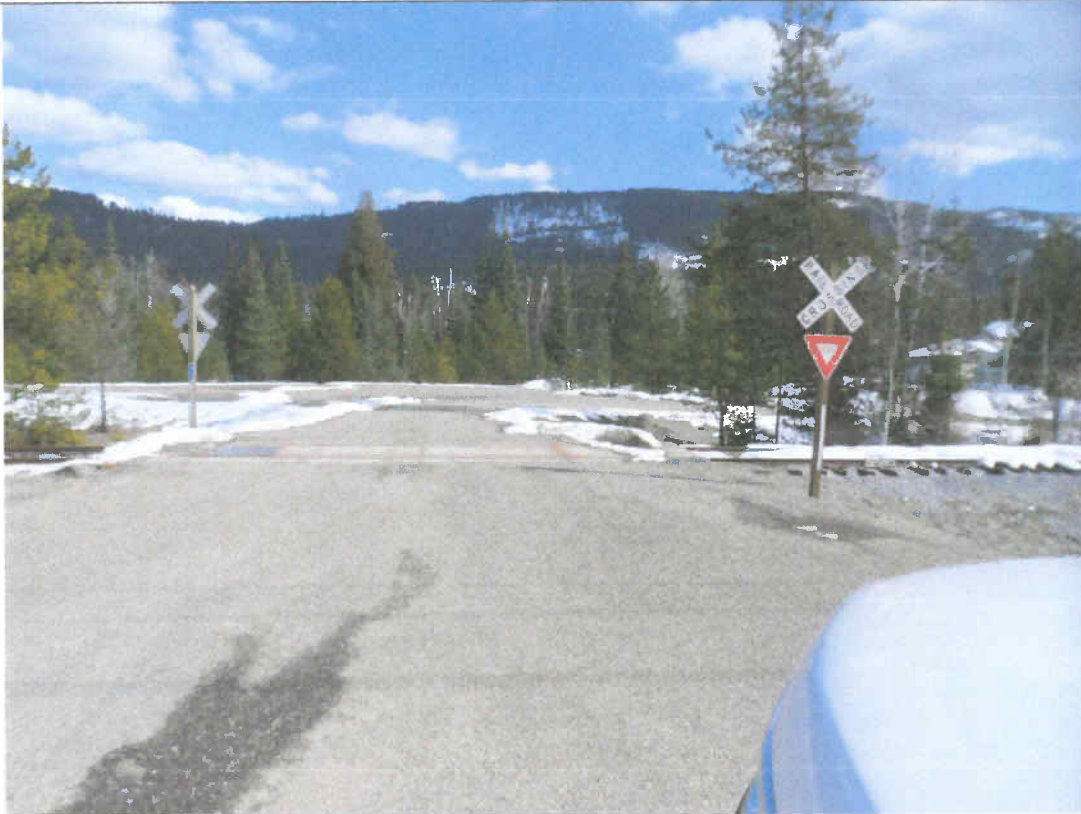
Crossing looking East from SR 20 to Ibbetson Drive
