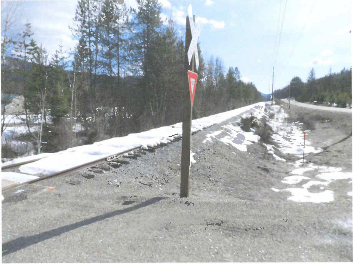
Ibbetson Drive Crossing looking South
