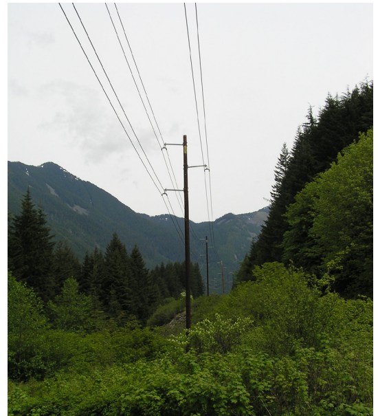
PSE cross-country transmission lines
