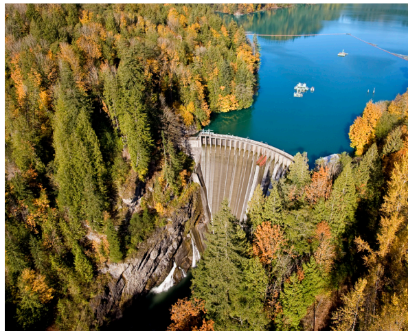
PSE's Lower Baker Dam in Skagit County
