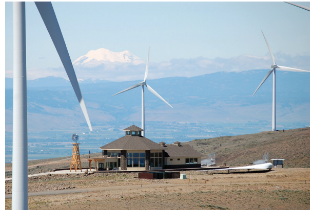
The Renewable Energy Center at PSE's Wild Horse Wind and Solar Facility in Kittitas County
