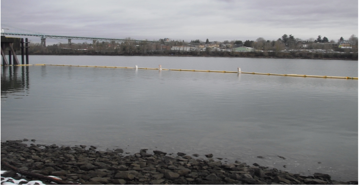
Photo 1 Centerline Oil Boom Placement from Dock to Dolphin with Three Mariner Warning Buoys at Pilot Cap Area (2/27/2023)
