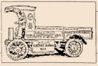
The above one-ton General Vehicle Co. truck, belonging to the Pacific Transfer Co., has been in service six months; has run 10.000 miles without one cent of repair coats. This truck is operated under our battery service system and runs 18 hours per day EVERY DAY and does the work of 3.12 to 4 texms of hornes, Over 4800 C. V. trackel on the some being in service 13 years.
