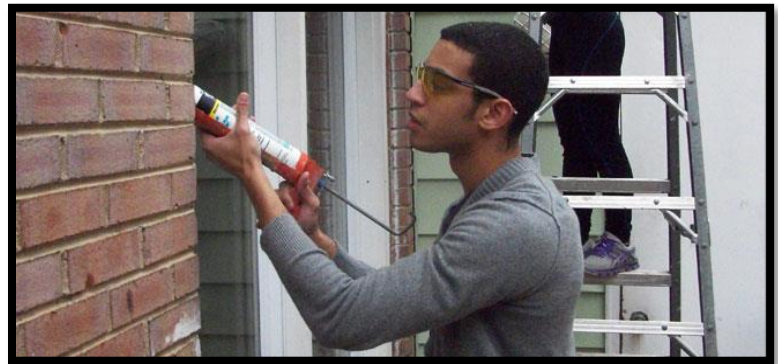
Weatherization of homes is easy and effective way to reduce energy use Source: Habitat for Humanity, Prince William County, VA
