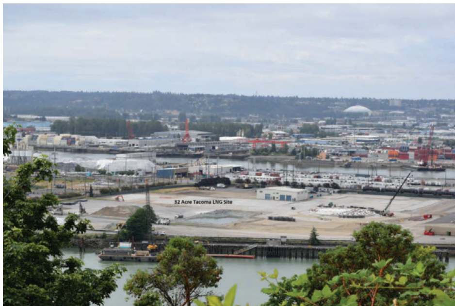
Figure 3 – Tacoma LNG Site, July 2017 (Looking South)
