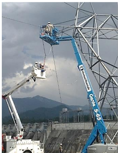
Transmission work at Noxon
