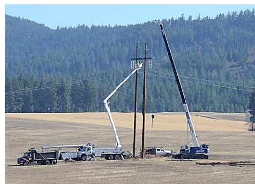
Avista rebuilding the Benewah-Moscow 230 kV line across the Palouse
