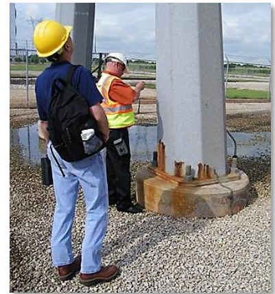
Steel Pole & Foundation Inspection
