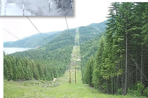
Below: Cleared right-of-way on the Cabinet – Rathdrum line
