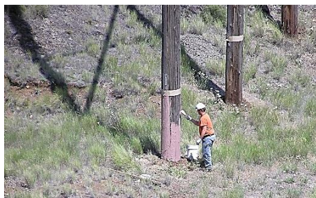
Replacing the fire retardant coating on the Lolo-Oxbow 230 kV line
