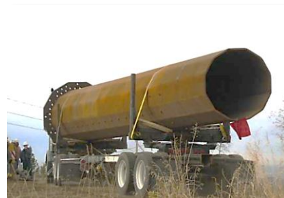
The 50 year old Beacon-Rathdrum line was rebuilt as part of the West of Hatwai Project
