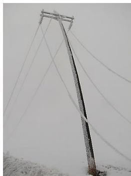
Snow & ice loading in Reardon breaks conductor and shatters a pole
