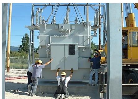
Crew setting distribution transformer at the Old Town Sub
