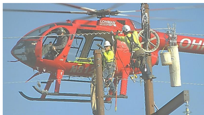
Working on the Benewah – Moscow 230 kV line
