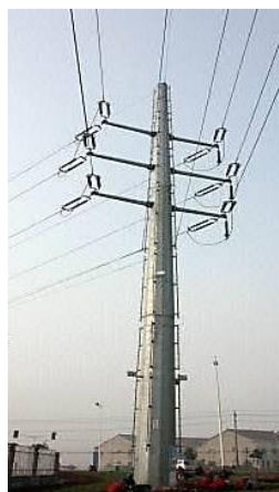
Above and right: Dead End Structures
