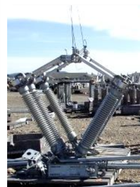
Right: Air switches waiting to be installed
