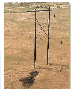
Above: Aerial inspection spots a lightning strike next to a pole
