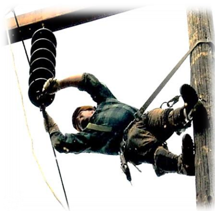
Replacing a broken insulator string is part of the Minor Rebuild program.
