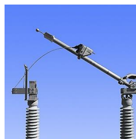
Above: Air Switch in open position
