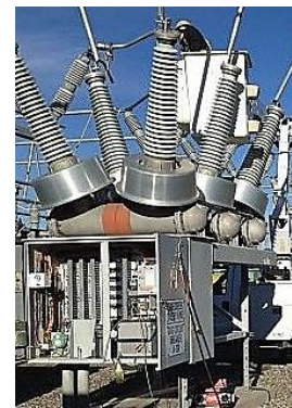
Avista High Voltage Circuit Breaker Undergoing Maintenance
