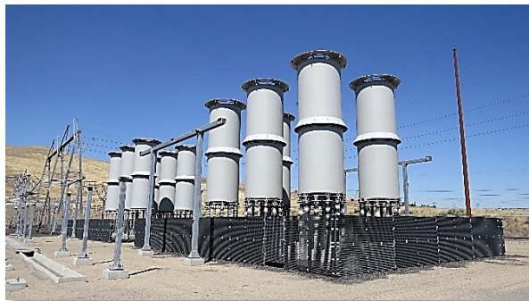
North Lewiston Reactors help regulate the voltage and reactive power in this area
