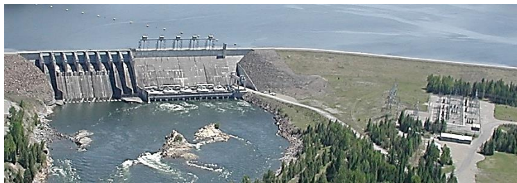
Noxon Rapids Dam with Switchyard on the Right
