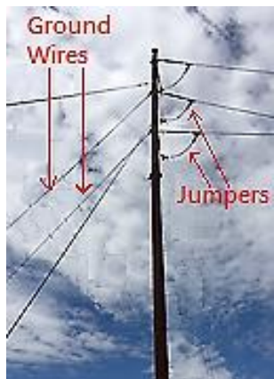
Above and right: Dead End Structures
