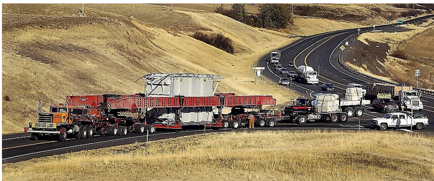
Dry Creek 230/115 transmission auto transformer making its way to Dry Creek Substation
