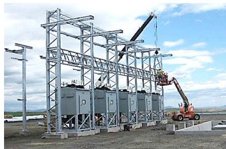
Upgrading Sunset Substation
