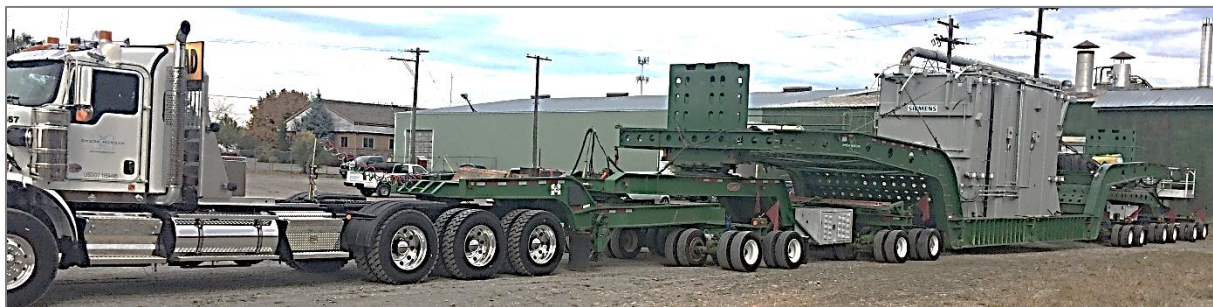
Today's auto transformer - the Pine Creek Auto Transformer being moved into position
