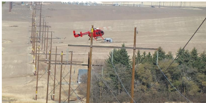
Using a helicopter to rebuild the 60 year old Benewah – Moscow Line
