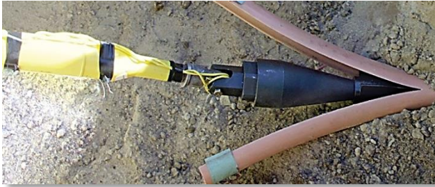
Split-and-pull pipeline replacement technique
