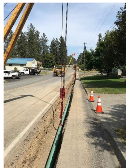
Gas Line Relocated for Road Work
