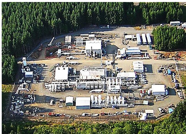
Jackson Prairie Underground Storage Facility
