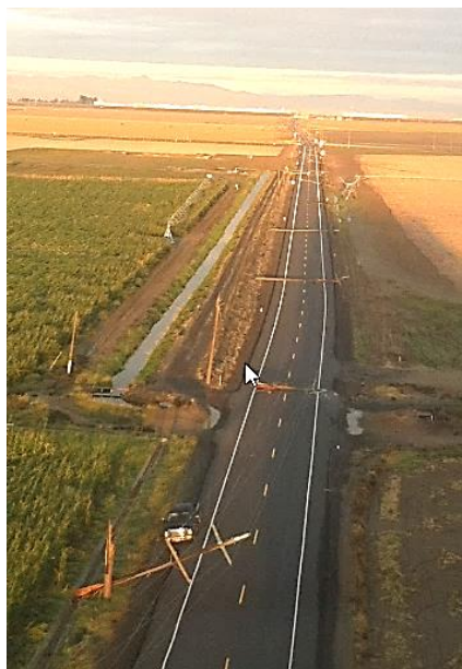
Powerful windstorms in the Othello area can cause major damage
