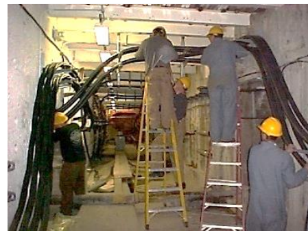
Working below the streets in the Downtown Network
