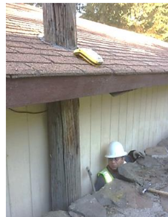
Crews face a variety of unique situations in inspecting wood poles
