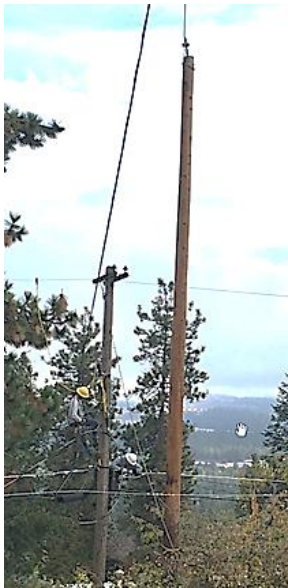
New pole being set with a crane
