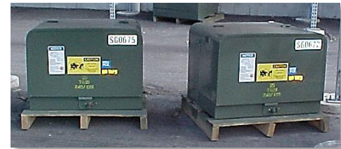
Above: Pad Mount Transformers awaiting installation Below: Submersible Transformers
