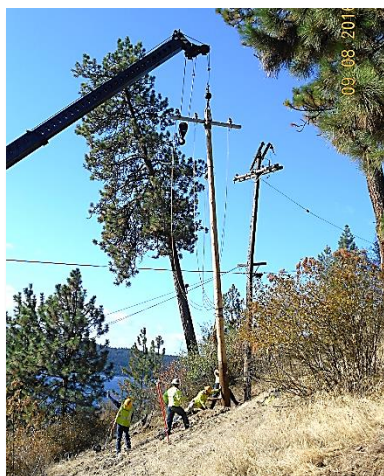
Above: A pole rots and fails Below: Replacing old pole with new (significantly straighter) pole Top Right: Pole hit by a truck Bottom Right: Wind storm causes a pole to split
