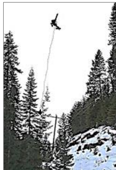
Grangeville’s terrain presents some major challenges. At times helicopters must be used to access lines.
