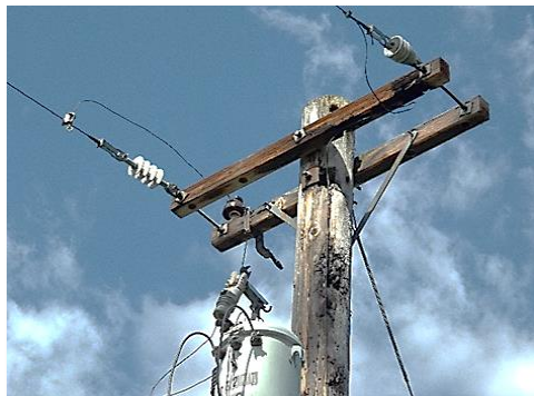
Above: Fire damaged pole Below: Broken crossarm
