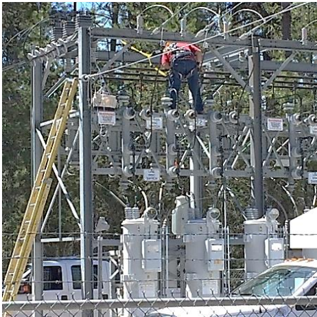
Working on a substation issue
