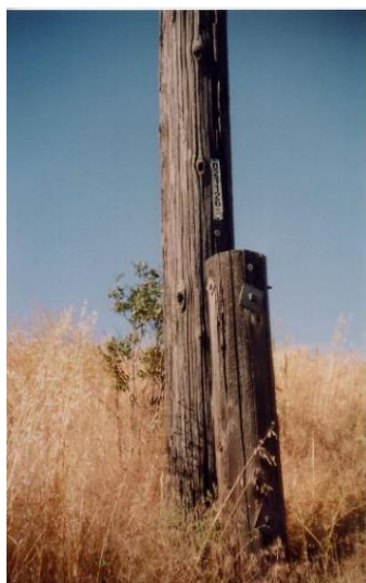
Stubbing a pole can add an additional 20 years or so to the life of a pole
