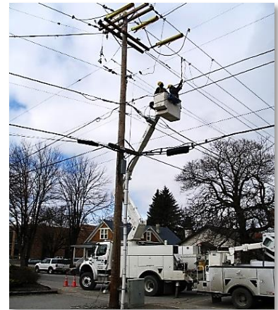
Spokane Linemen deal with the complexity of multiple foreign utilities located on their poles
