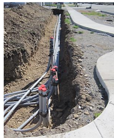
Installing Underground in Coeur d’Alene
