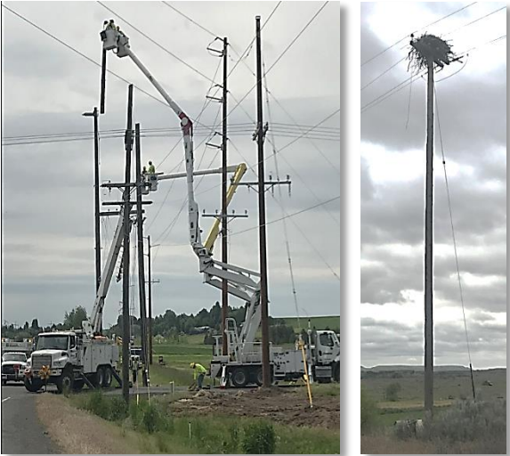
Left: moving poles and lines for a county road project
