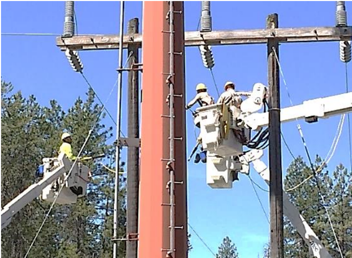
Deer Park Crew repairing transmission
