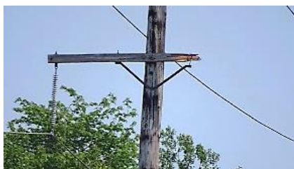
Above: Fire damaged pole Below: Broken crossarm
