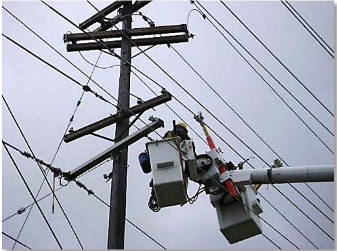
Overhead distribution work
