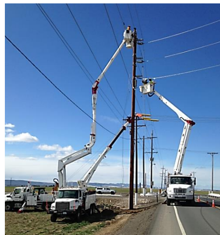
Upgrading Othello transmission lines
