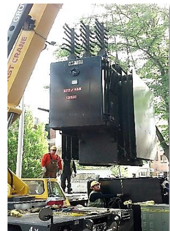
Placing a Pad Mount Transformer
