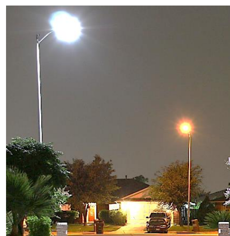
LED (left) vs. Sodium (right)
