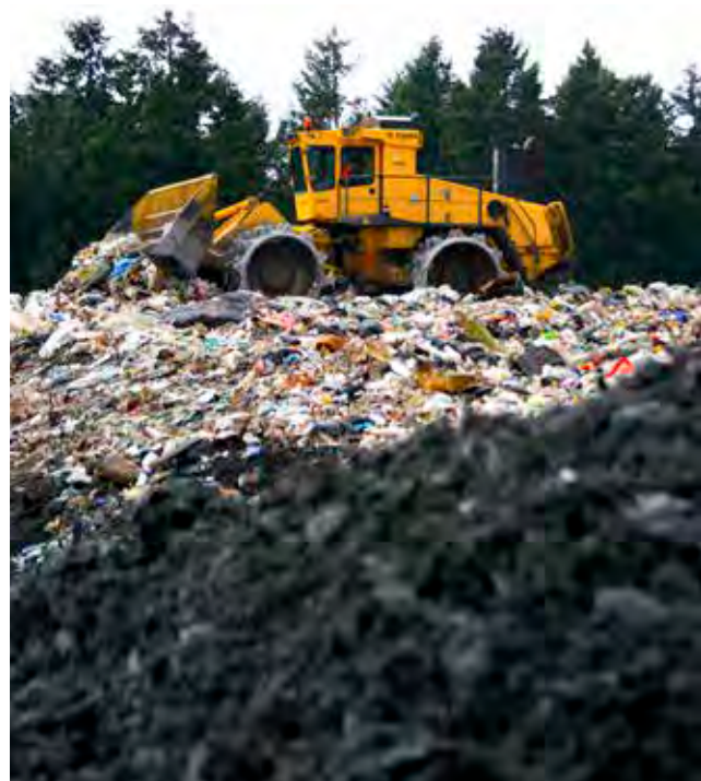
A bulldozer compacts waste at the Cedar Hills landfill
