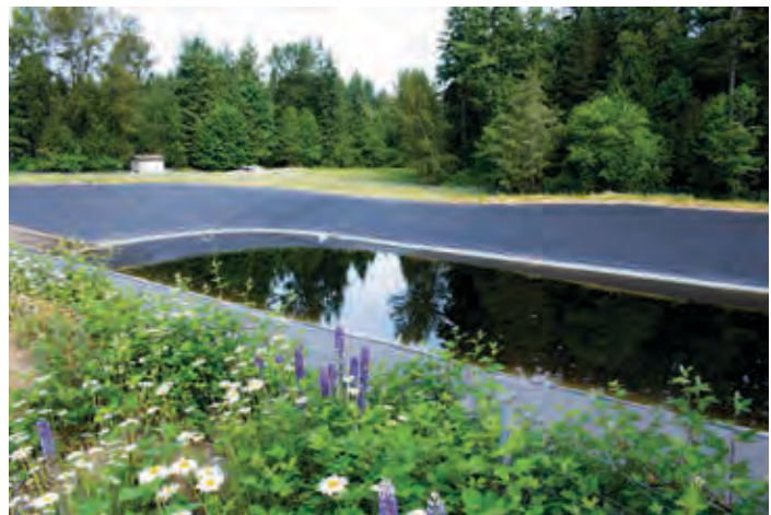
A stormwater pond at the Cedar Hills Landfill II is part of the infrastructure paid for by the Facility Improvements Account
