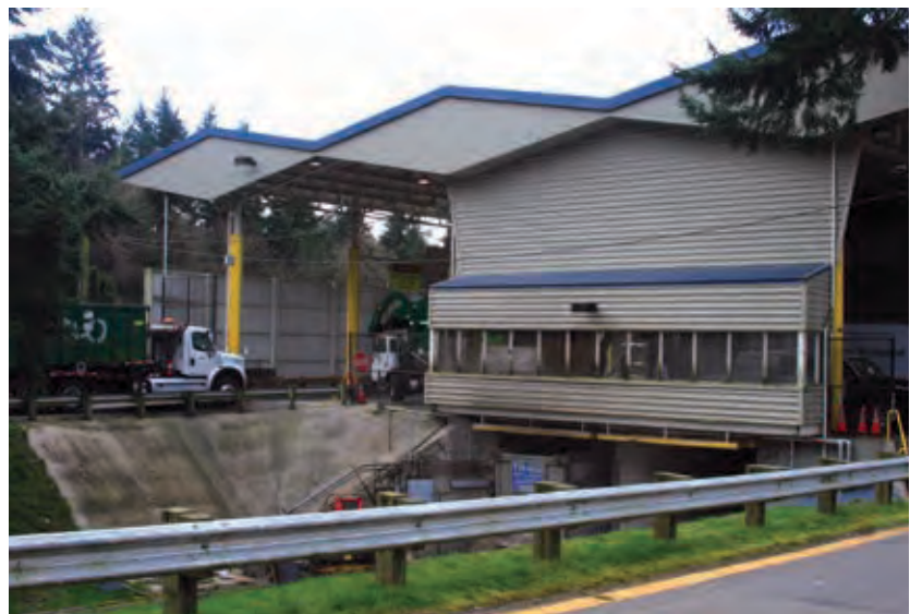
The roof at the Houghton Transfer Station was raised in 2012 to accommodate larger trucks
