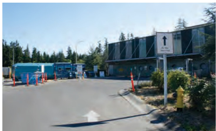
The Vashon Recycling and Transfer Station
