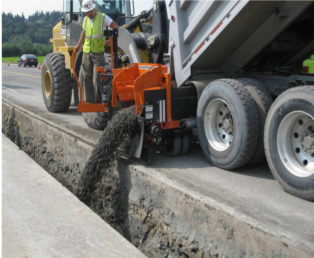
Figure 4-4: Kent Black Diamond Phase II Project, 16-Inch Diameter Supply Pipeline, In-Service 2009
