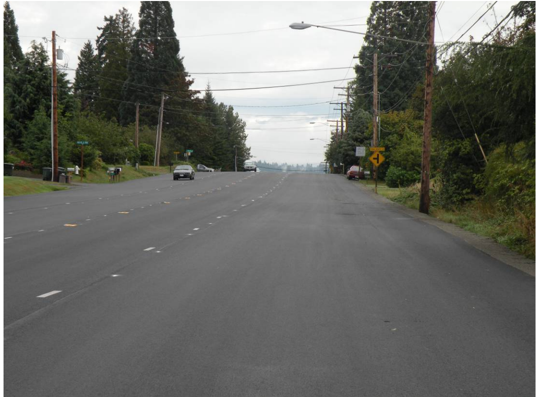
Figure 4-3: Kent Black Diamond Phase II Project, 16-Inch Diameter Supply Pipeline, In-Service October 2009
