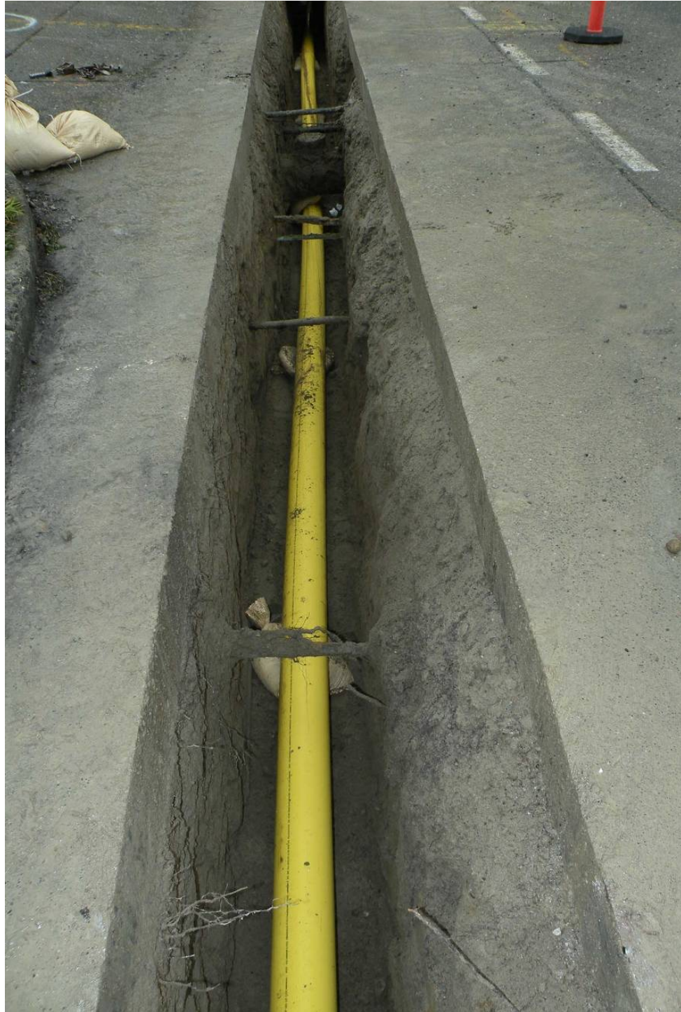
Figure 4-5: 6501 Beacon Ave S, 6-Inch Bare Steel Main Replacement, In-Service Expected 2010
