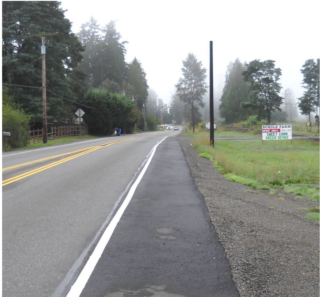
Figure 4-1: Orting Phase I Project, 8-Inch Diameter Supply Pipeline, In-Service 2007
