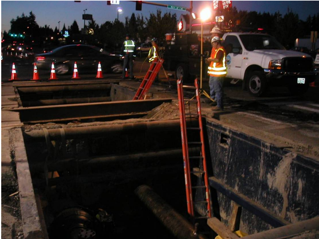
Figure 4-8: Lynnwood Valve Replacement, In-Service 2007
