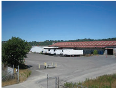
View North of the Tideflats Station
