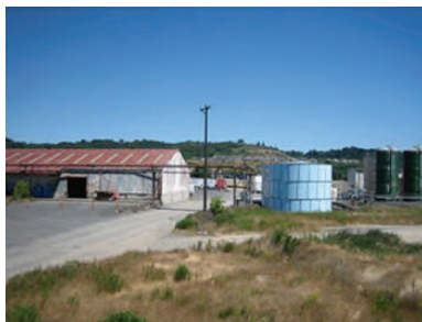
View Northeast of the Tideflats Station
