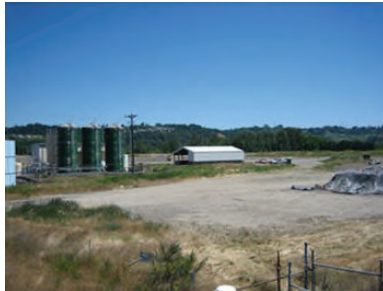
View East of the Tideflats Station
