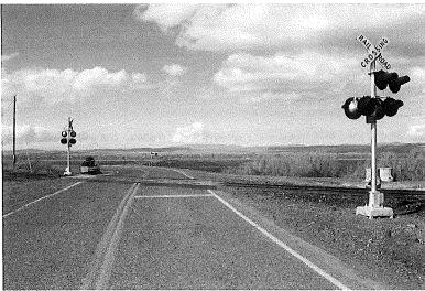
funded by the WUTC and installed in 2013.<sup>55</sup> While there are turns near the crossing, the advance LED warning signs alert drivers in advance of the turns, and the tracks are in the middle of a 400 foot straightaway.<sup>56</sup> As with the Myers Road crossing, the visibility at the South Track Road crossing is excellent in each direction, from each approach.<sup>57</sup>
