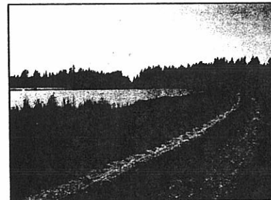
Dike 14 at Printz Basin
