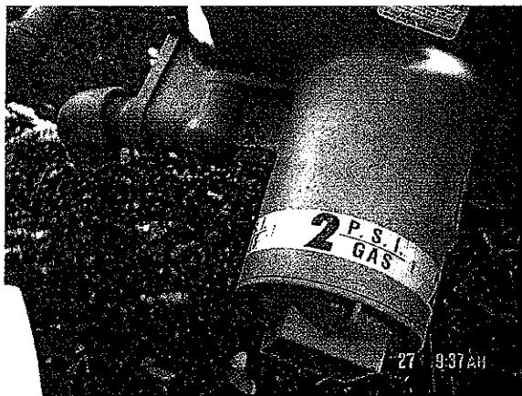
Figure 3. Meter #743434: Corrected regulator vent.
