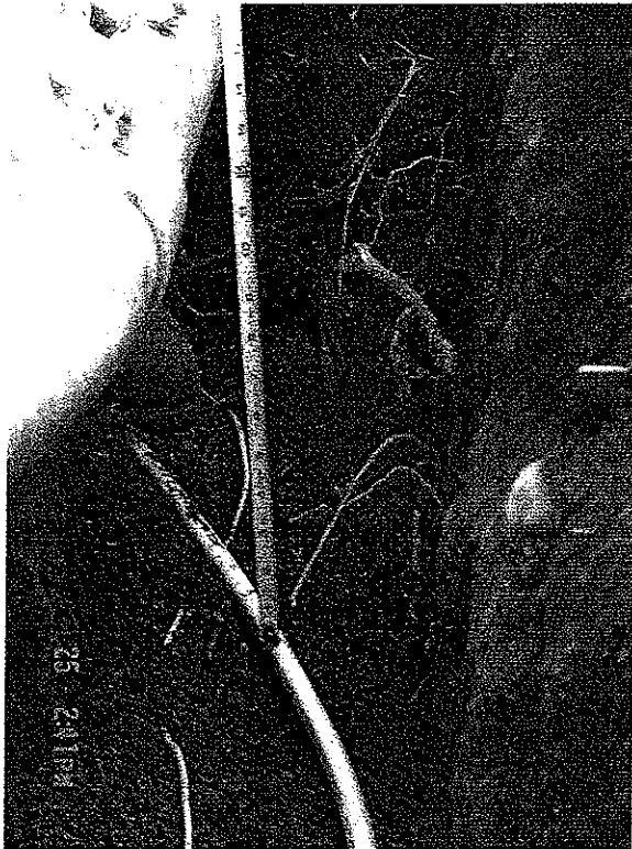
Figure 7. 9117 NE 77th Street, Vancouver: Depicts approximately 15-inch separation between gas line and other utilities.
