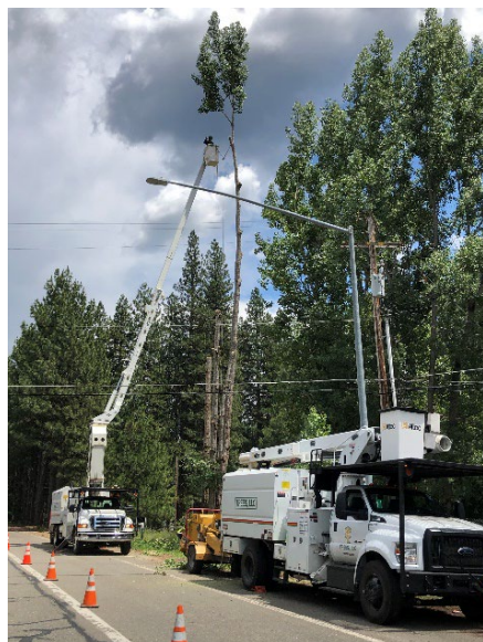
Figure 33: High-Risk Tree Removal
