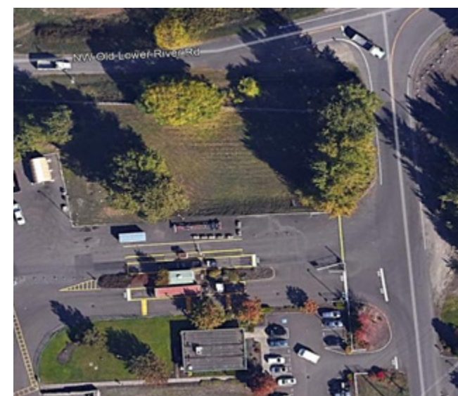
Figure 6: West Van Entrance and Scale Complex
