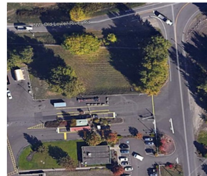
Figure 5: West Van Entrance and Scale Complex
