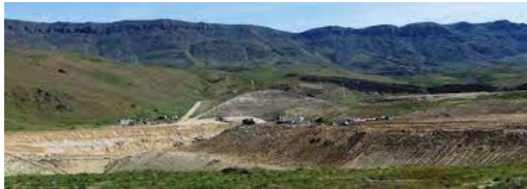
Figure 5-2. Greater Wenatchee Regional Landfill
