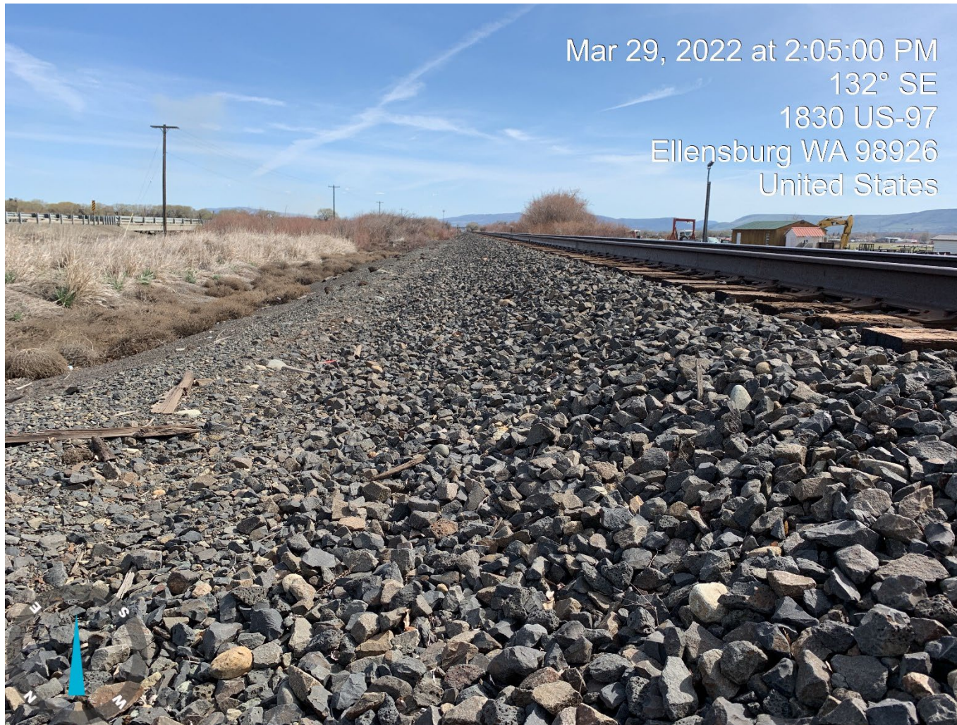
Ellensburg MP 2.5 steep roadbed at incident location
