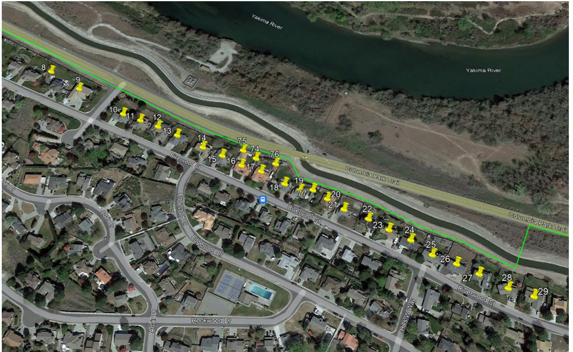
Figure 3: Section of the proposed Richland HP Lateral showing its proximity to buildings 8-29 & 74-77 within the 100-foot boundary.
