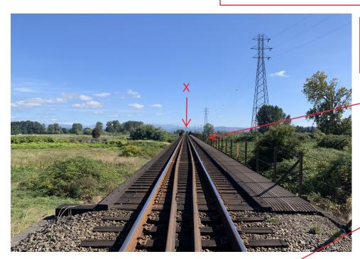
Sight distance to the east is limited due to the arch of the bridge deck. This is the direction the train was headed. Incident location is marked with an X.
