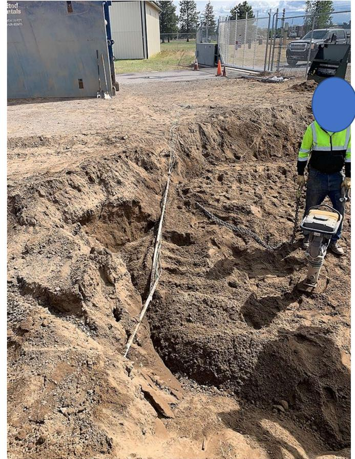
Locates coming into back of Power Box but no locates going out of the power box.
