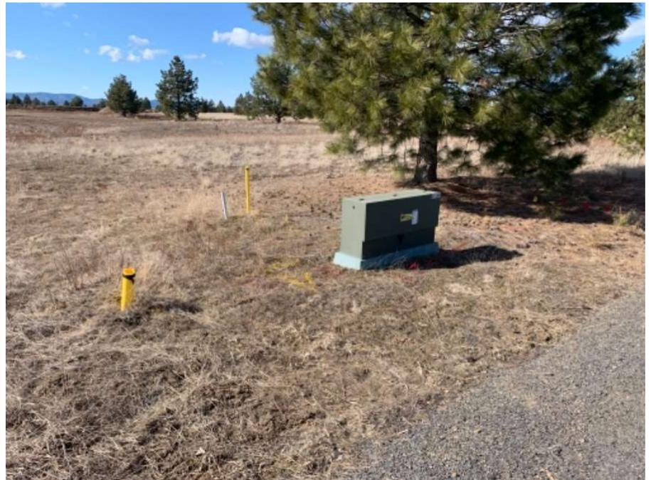
The Northern section of the project had a few old flags laying in the grass and markings around power boxes but no crossings or locates between the power boxes. Because of the missing locates another Locate ticket was called in.
