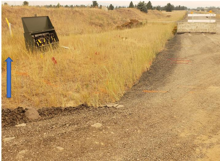
On 8.5.2021 the Locate ticket called in on 8.2.2021 went live and a power line was struck. There was three older locate marks that were not refreshed on the new locate coming out of the power box with an arrow towards the water tower.
