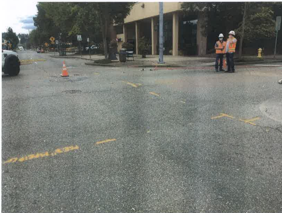
1424 looking SW, locates after incident show PSE assets-orange cone is leak location
