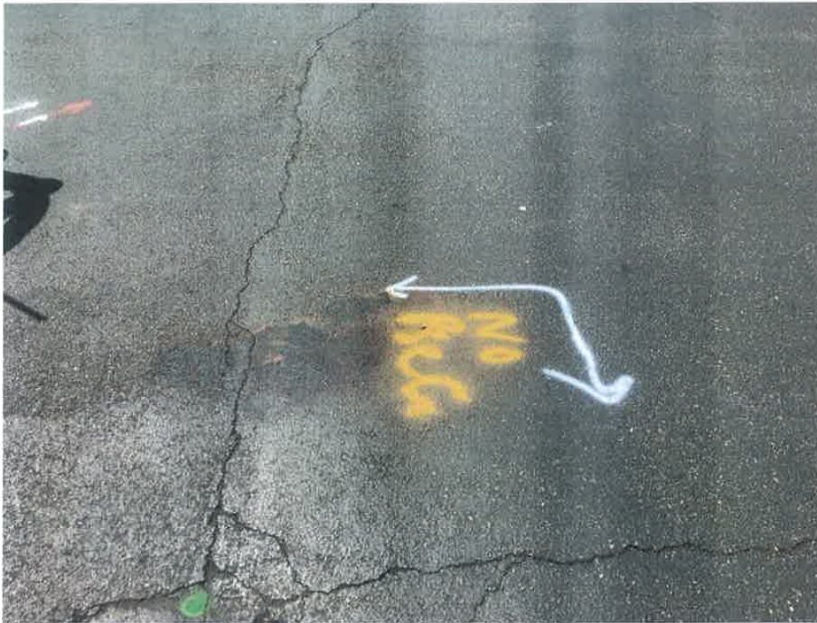
1351-looking S in US Bank Parking lot-NO PSEG marking by ELM locator, SEFNCO white locate paint
