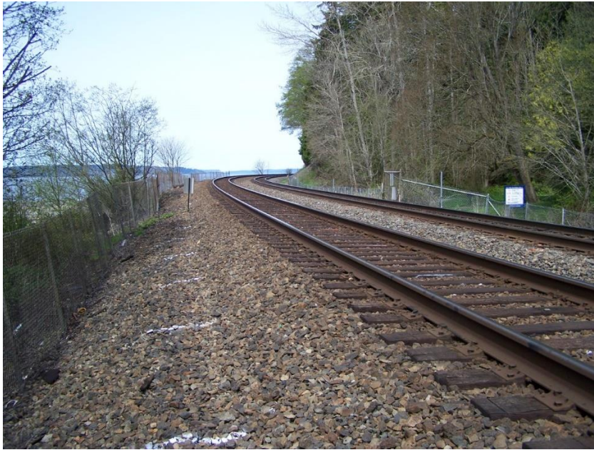
Photo 13: Railroad curvature reduces sight distance for trespassers and adjacent bluff dampens sound of train approaching
