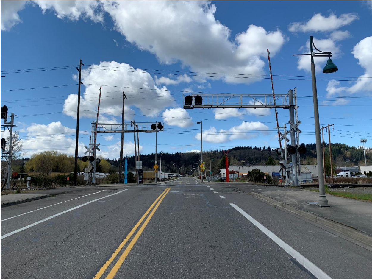
TR-200848 (2) Facing East Toward Accident Site. Photo Taken by Andrew McMahon on 04/08/2021.
