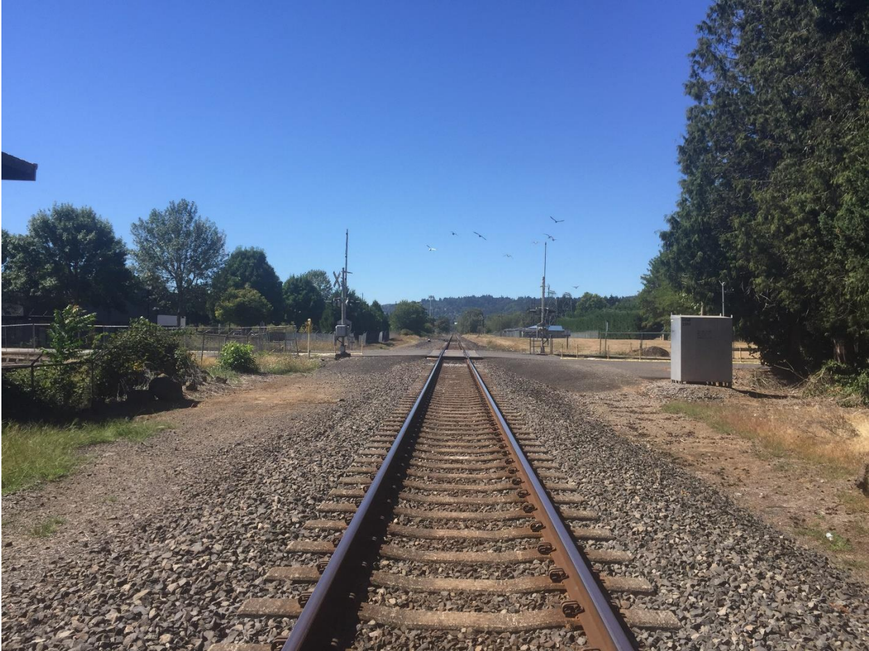
TR-190786 (1) Facing West Toward Accident Site. Photo by Andrew McMahon on 09-03-2020.
