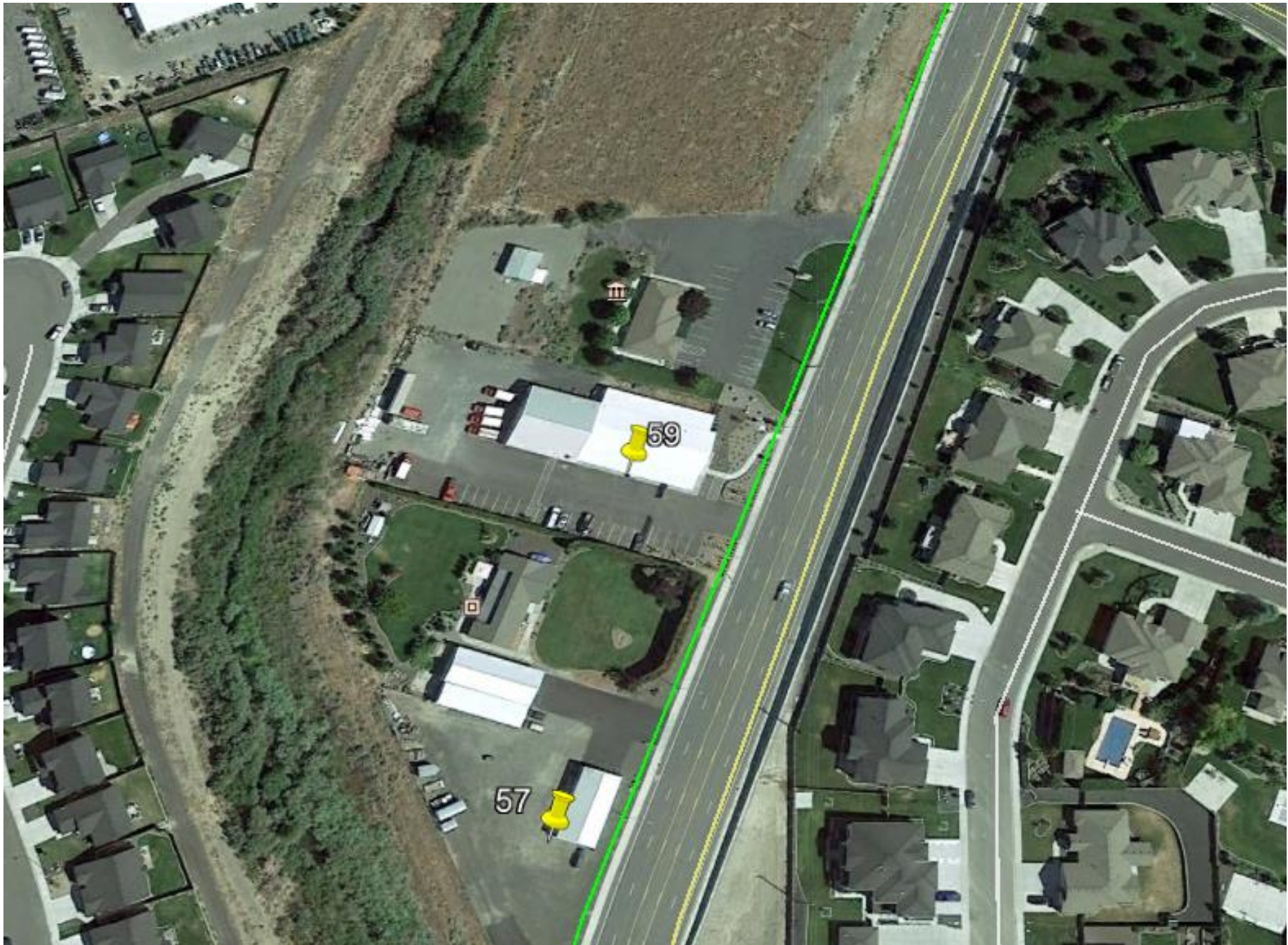
Figure 6: Fifth section of Southridge HP showing buildings 57 & 59 within the 100-foot proximity to the pipeline.
