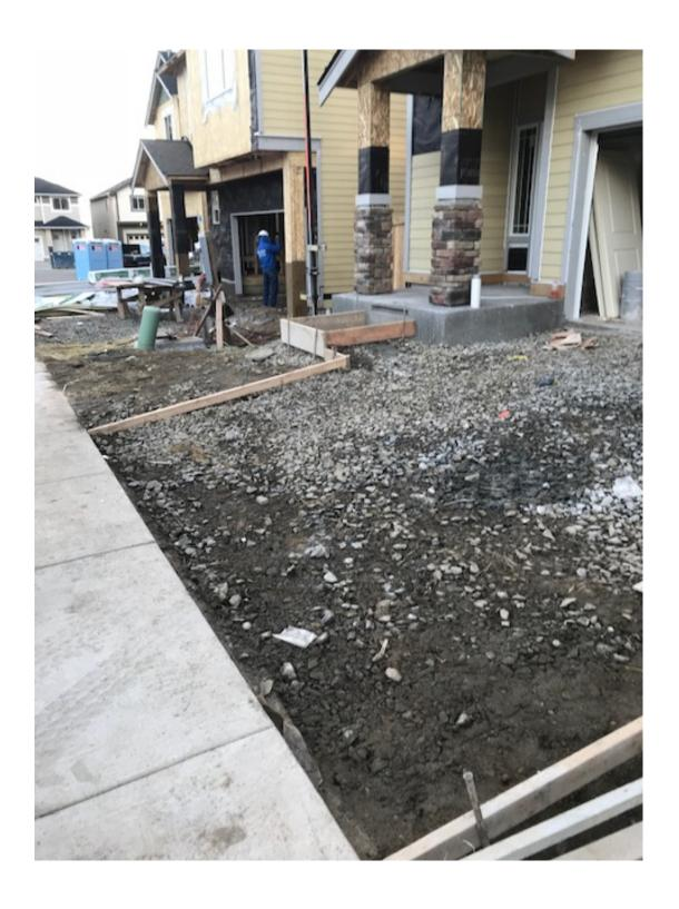
• As evidenced by this series of pictures there are stakes inserted in the ground even though they did not have a valid locate ticket
