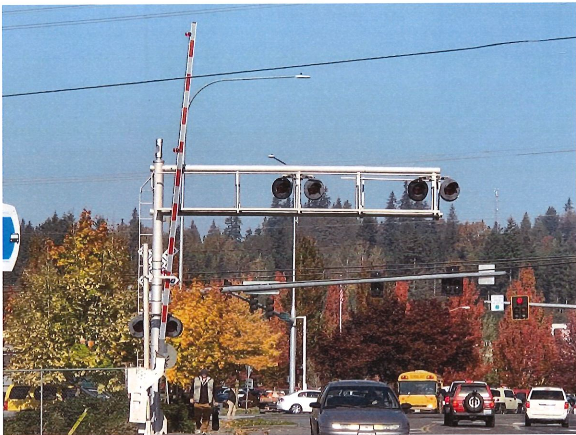
Photo 3: Northbound view on Kelsey St. of southbound gate for Crossing 084565X.
