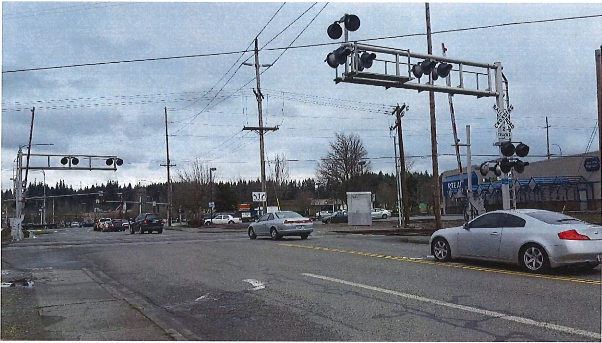
Photo 1: Northbound view on Kelsey St. of Crossing 084565X with gates raised.
