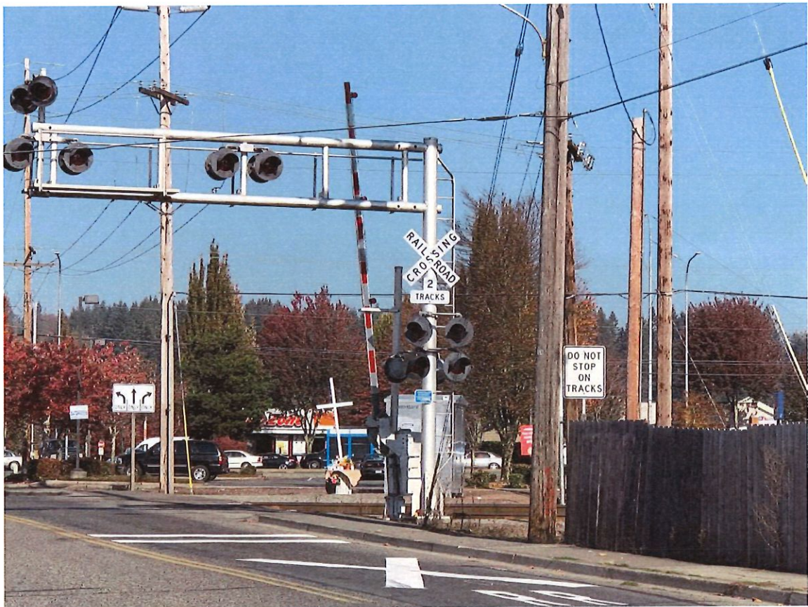
Photo 3: Northbound view on Kelsey St. of northbound gate for Crossing 084565X.
