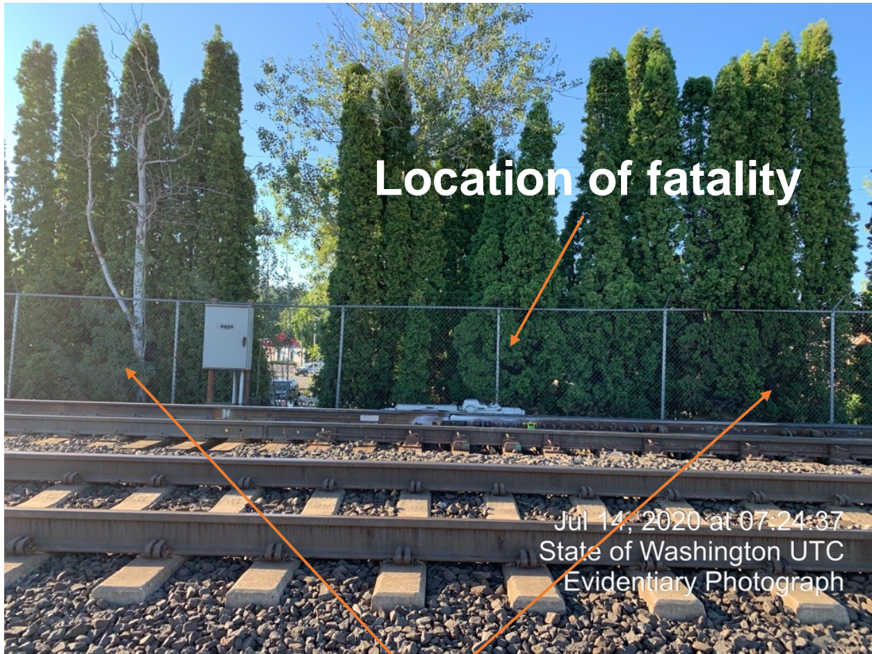
Photo showing fencing that restricts ability to use railroad property for direct passage
