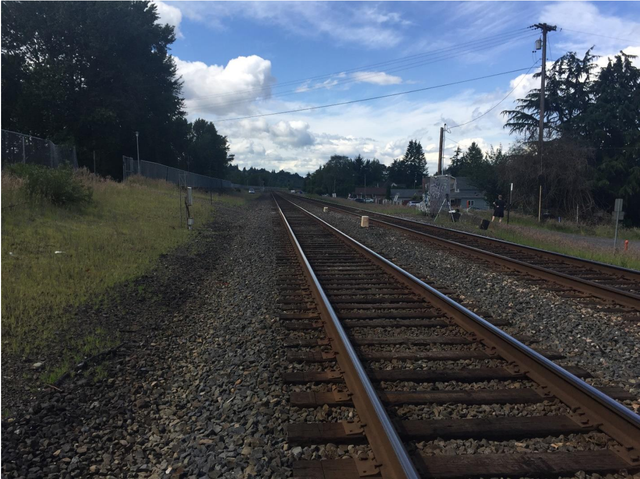
TR-180741 (1) Facing North Toward Accident Site. Photo Taken by Andrew McMahon on 06/10/2020.
