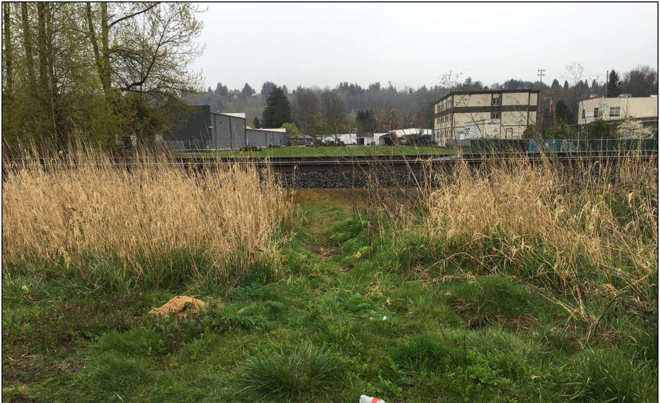
Informal trespassing pathway 0.33 miles north of James Street. Trains travel at speeds up to 79 mph with no warning devices at this location to alert people to their presence.
