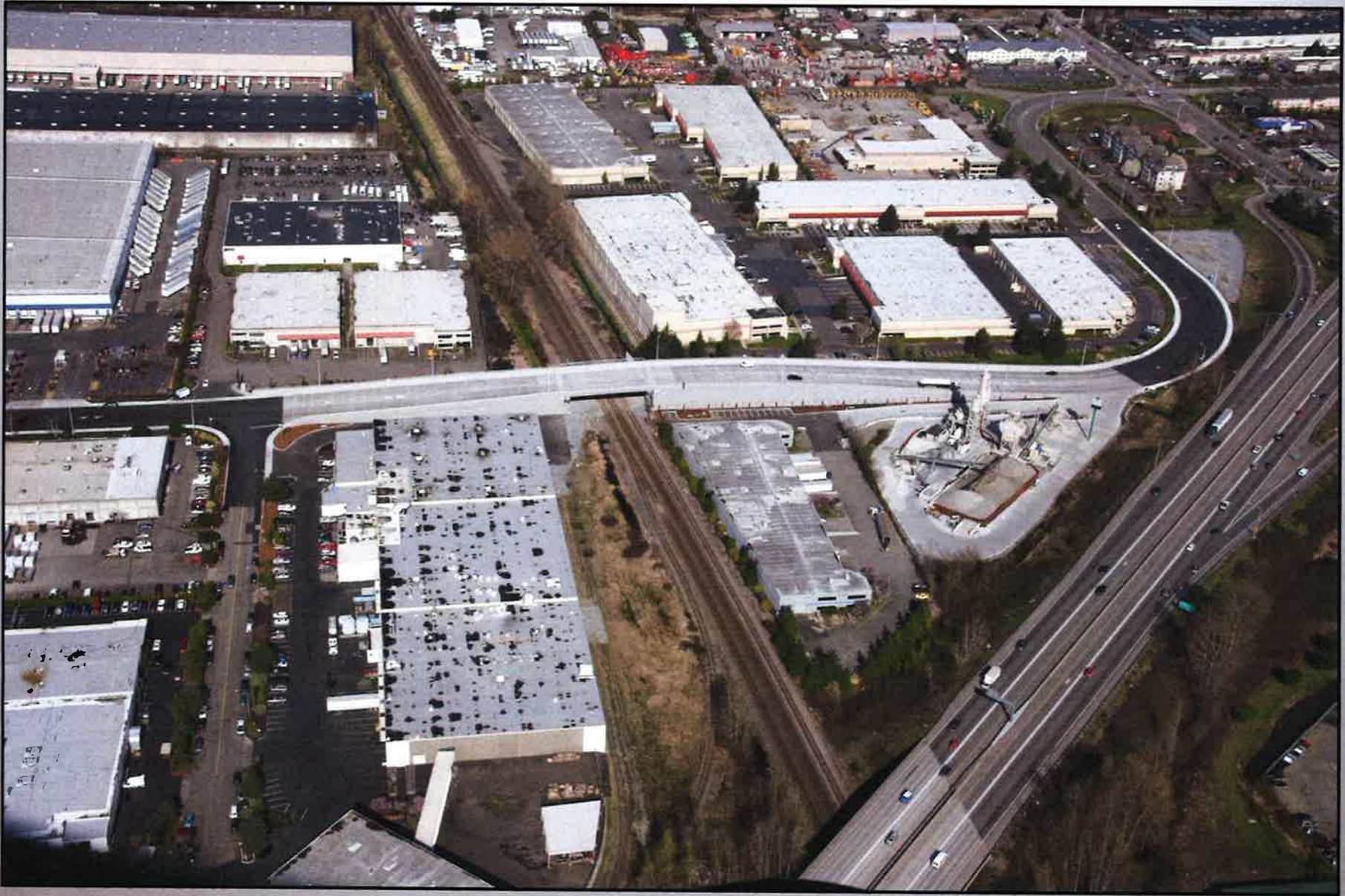
S. 228 th St. BNSF Grade Separation
