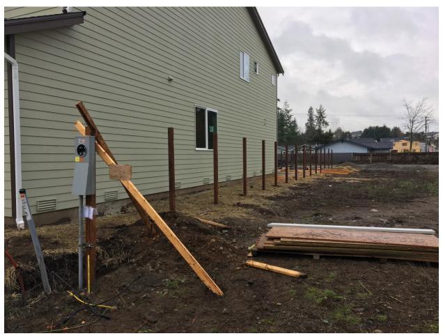
It is obvious that the fence line is located in the proximity of the gas and electric utilities. No locates on the ground.
