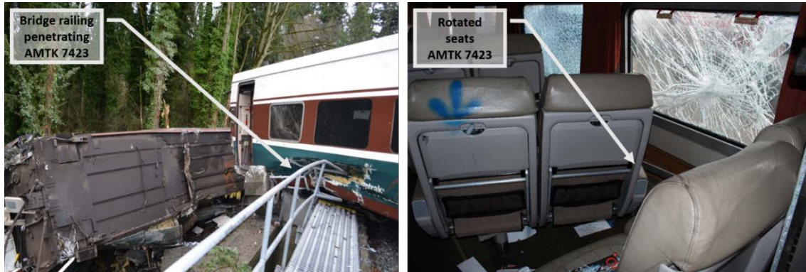
Figure 31. Bridge railing penetrating AMTK 7423 and displaced passenger seats.
