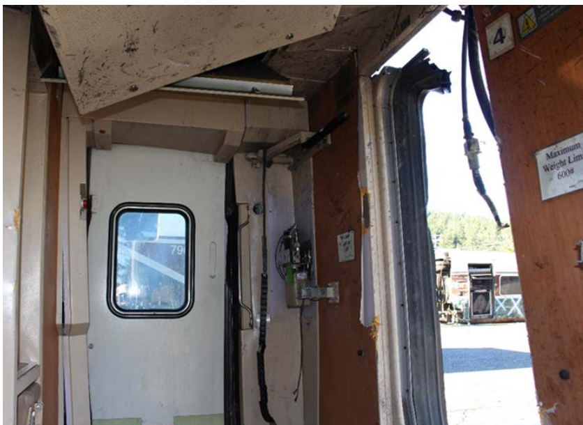
Figure 34. Photograph of missing wheelchair lift and damage to AMTK 7504 (7).
