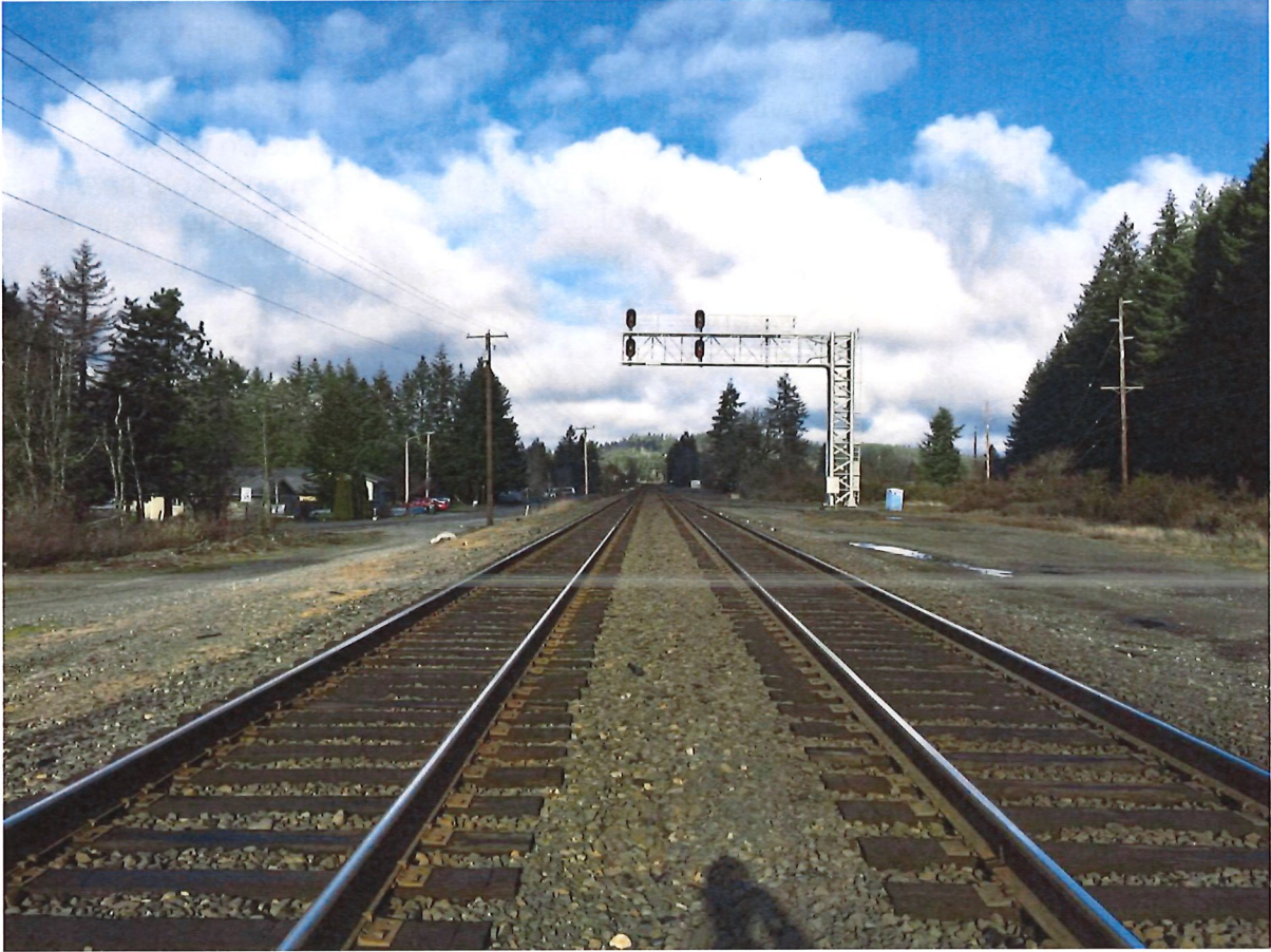
TR-170876 (1) Facing North Toward Accident Site. Photo Taken by Andrew McMahon on 12/27/2018.
