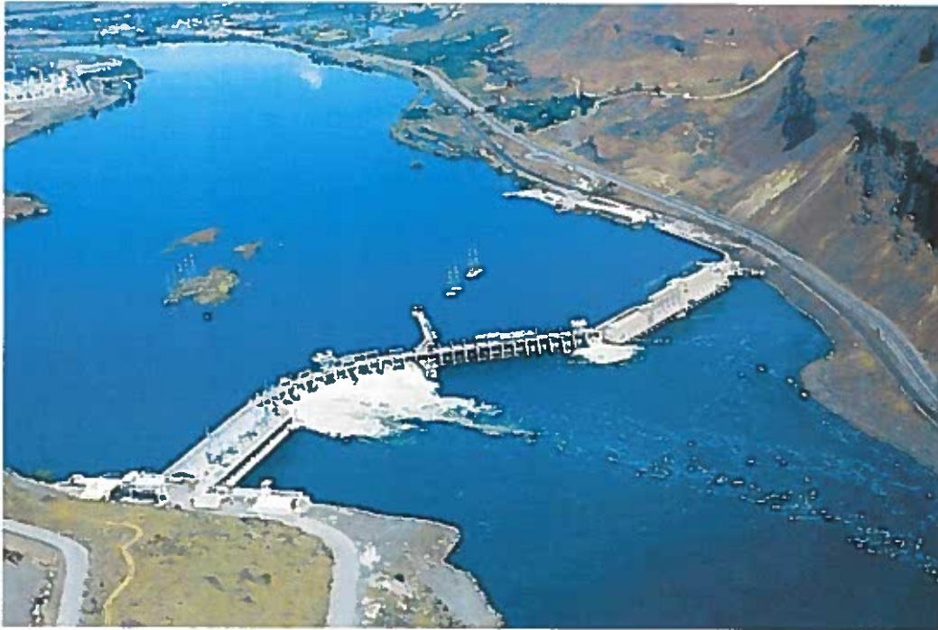
Photo 2: Rock Island Dam
