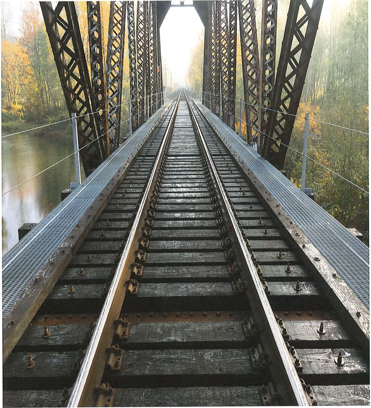
View looking East
