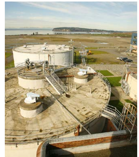
An anaerobic digester at the Chambers Creek Regional Wastewater Treatment Plant is used for breaking down organic material
